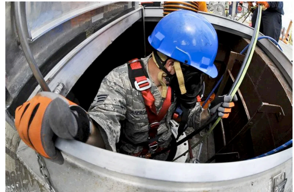
Figure 1. Confined Space Entry
